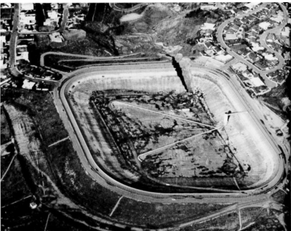
FIGURE 5 A breached reservoir in Los Angeles, California, that reflects unfortunate interplay between man and the local geologic scene. This facility was constructed across the surface traces of several small faults that appeared to be inactive. Movements of several inches occurred along at least one of these faults, however, and ultimately led to failure of the reservoir wall and catastrophic flooding of a nearby residential area in 1964.
