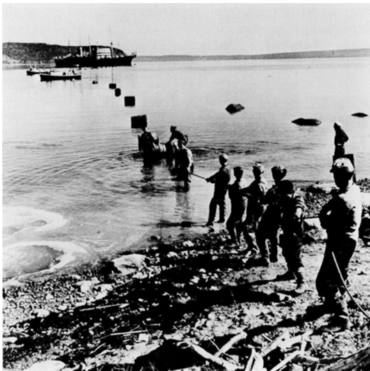
FIGURE 2 In 1955, the first cable to deliver high-quality telephone service was laid between North America and Oban, Scotland. Here it is being pulled ashore at Clarenville, Newfoundland. It was floated on shallow steel drums, loaded into a trench, and routed to the shore station. The cable was 1,940.8 nautical miles long and began operation at 11 A.M., EST, on September 25, 1956.
